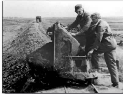
Spoil being tipped to build up the sea wall at Freiston Shore, as seen in the early 1970s.
